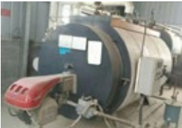
Air supply fan for boiler
